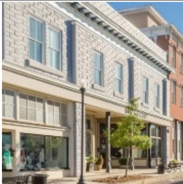
a & b. This building at least one (1) modulations in the façade plane.
