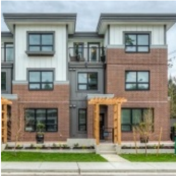
a. The building provides detailing that transition the façade material changes.
